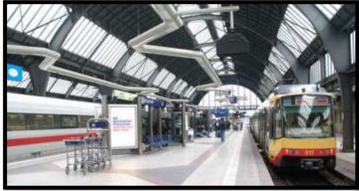
Figure 2-2: High-speed rail (left) sharing platform with interurban train (right) in Karlsruhe, Germany, an example of integration Source: Mundus Gregorius via Flickr
